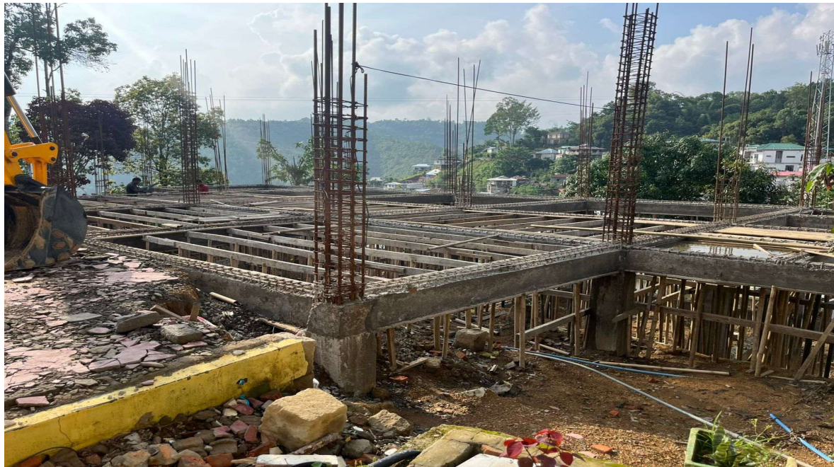
Ongoing construction of Champhai UPHC
